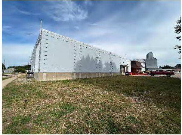
Front of Plant
