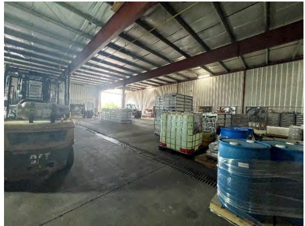
Interior Plant Live Hold/CAS Area
