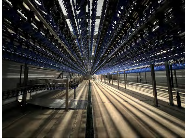
Air Chill Room
