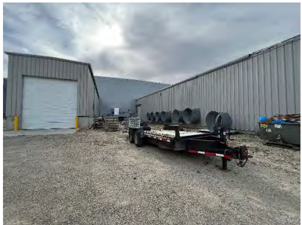
Rear of Plant
