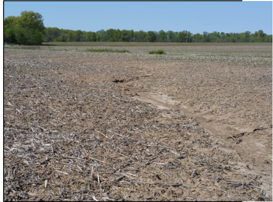
Figure 8: This ephemeral gully was found on the same producer's tract as Figure 7 and made the producer noncompliant.
