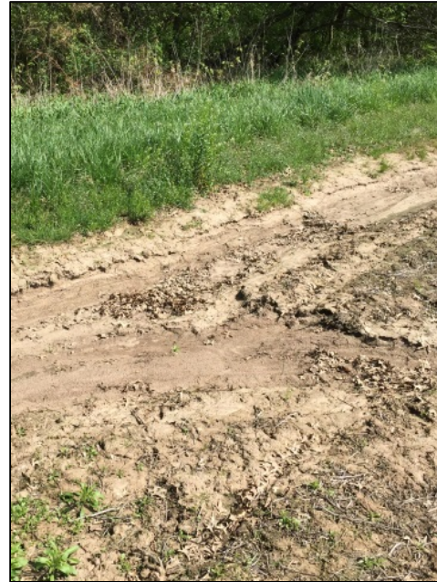
Figure 4: According to Missouri State officials, if soil is being displaced, the producer would be considered noncompliant, regardless of whether the soil stays on the producer's field.
